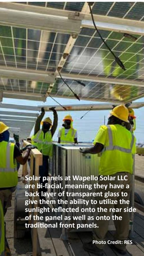
Solar panels at Wapello Solar LLC are bi-facial, meaning they have a back layer of transparent glass to give them the ability to utilize the sunlight reflected onto the rear side of the panel as well as onto the traditional front panels.
