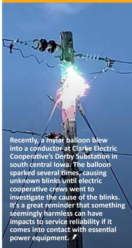
Recently, a mylar balloon blew into a conductor at Clarke Electric Cooperative’s Derby Substation in south central Iowa. The balloon sparked several times, causing unknown blinks until electric cooperative crews went to investigate the cause of the blinks. It’s a great reminder that something seemingly harmless can have impacts to service reliability if it comes into contact with essential power equipment. ⚡
