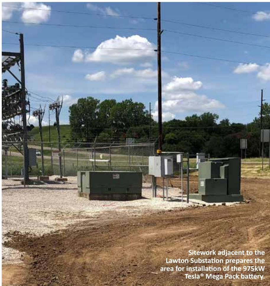
Sitework adjacent to the Lawton Substation prepares the area for installation of the 975kW Tesla® Mega Pack battery.
