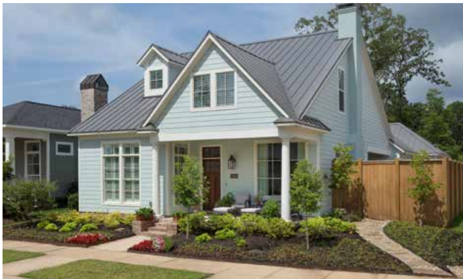
Photo Credit: McElroy Metal
