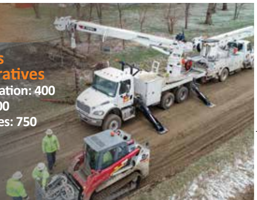
Photo: Northwest Iowa Power Cooperative
