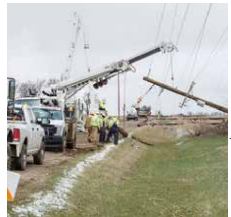
Photo: Northwest Iowa Power Cooperative
