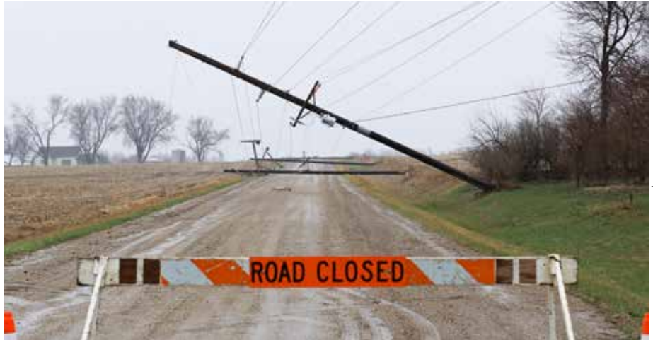
Photo: Northwest Iowa Power Cooperative
