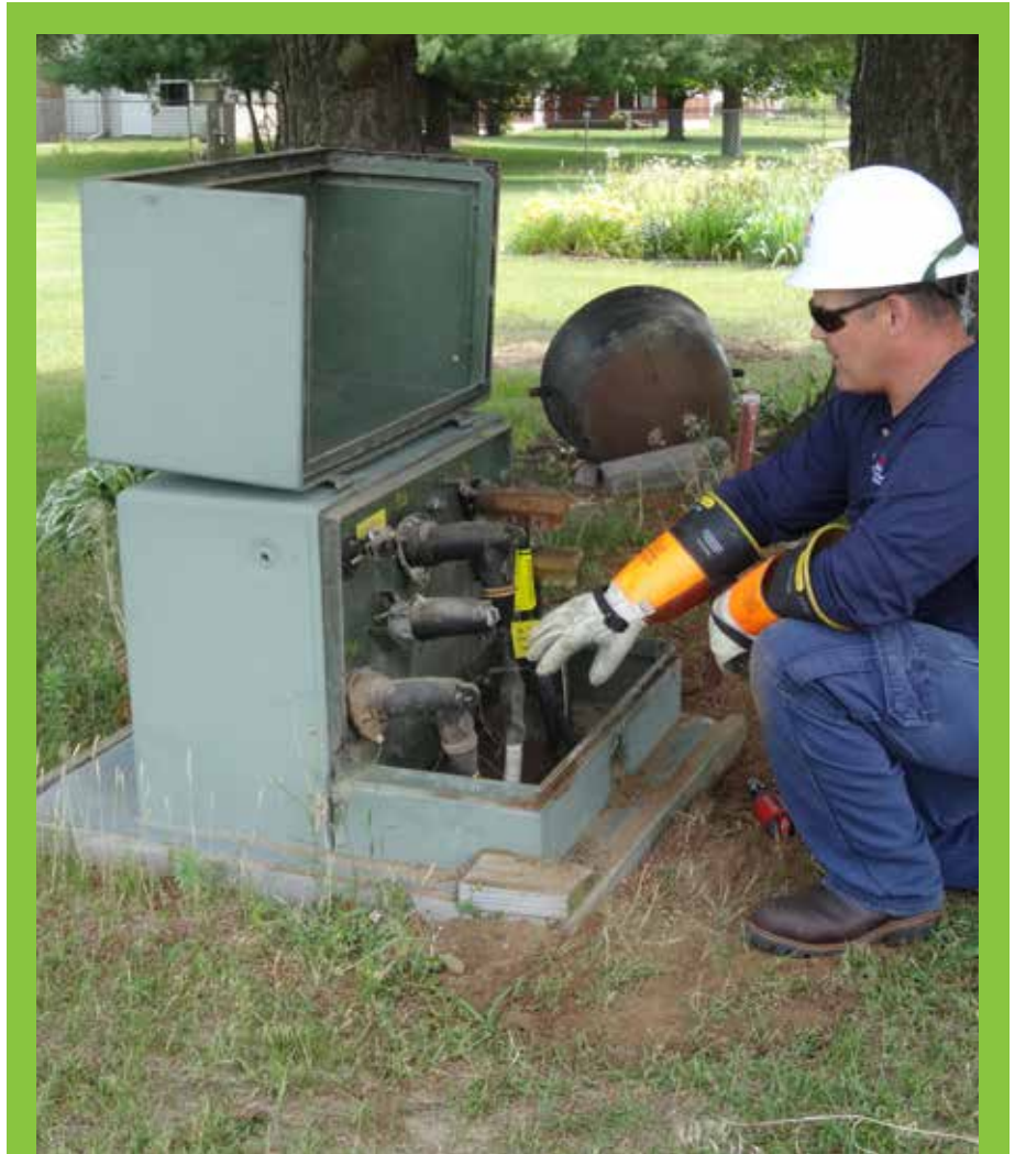
Pad-mounted transformers route large amounts of electricity and you should avoid them. Only professional lineworkers and crews should be near them.
