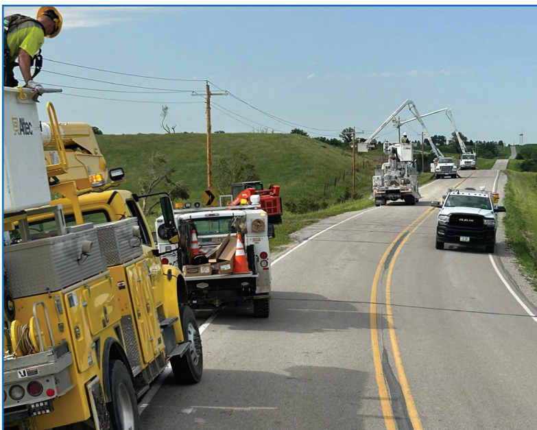
SWIAREC and Chariton Valley crews working on restringing line
